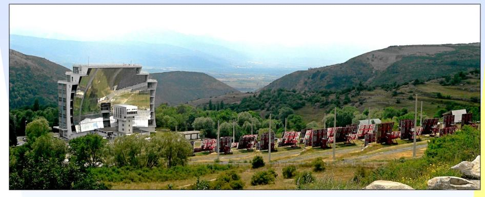
The solar furnace at Odeillo in the Pyrénées-Orientales in France can reach temperatures up to 3,500 °C (6,330 °F).
