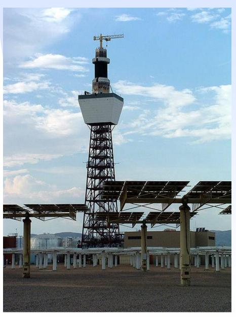
"Within the receiver the concentrated sunlight heats molten salt to over 1,000 °F (538 °C). The heated molten salt then flows into a thermal storage tank where it is stored, maintaining 98% thermal efficiency, and eventually pumped to a steam generator."
