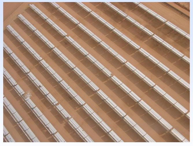
Nine solar power plants totaling 354 MW – the largest solar thermal plant in the world. At night, the turbines burn natural gas. The facilities have a total of 936,384 mirrors; lined up, the parabolic mirrors would extend over 229 miles (369 km). An automated washing mechanism is used to periodically clean the parabolic reflective panels.
