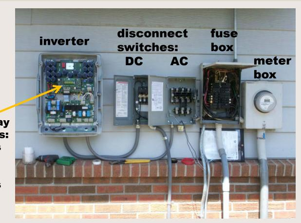
display shows: watts kwh volts hours etc.
