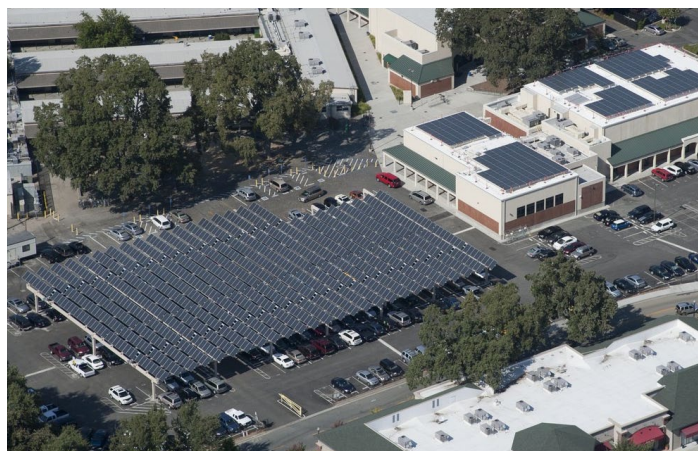
Commercial photovoltaic installation on commercial building and parking shade structure in San Ramon, California
